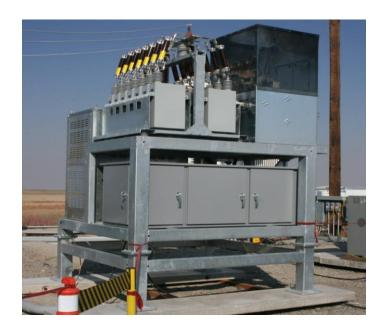
Figure 1 - Photo of the  $SolidGround^{TM}$  Transformer Neutral Blocking System
